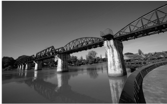
Figure 1 Bridge over the River Kwai
