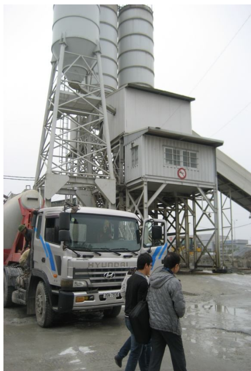
Figure 1 Ready-mix Batching Plant, TRANSMESCO
