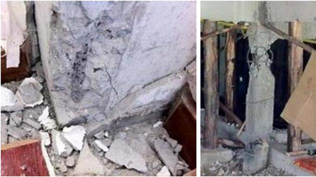
**Figure 1** Failure of RC columns during Mae Lao earthquake [1]
