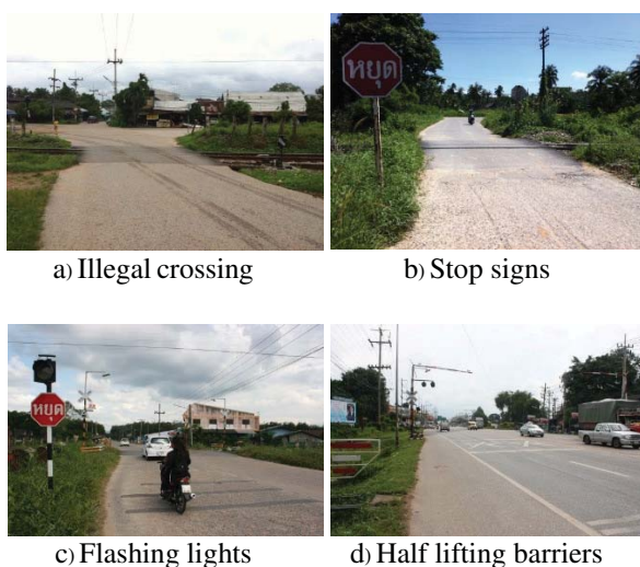
Figure 2 HRGC Traffic warning devices
